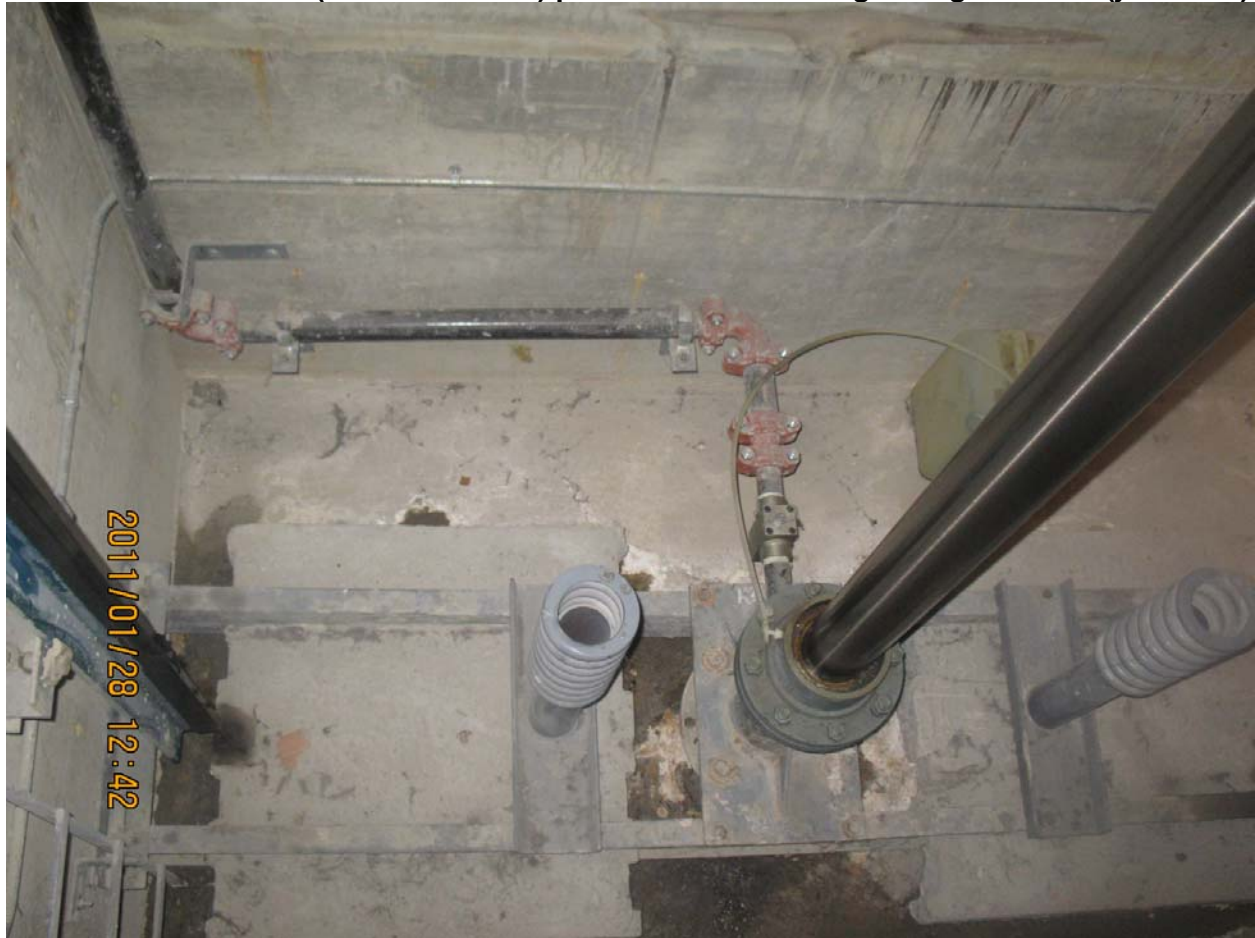
Photo 12 – Bottom of elevator car and jack plunger
