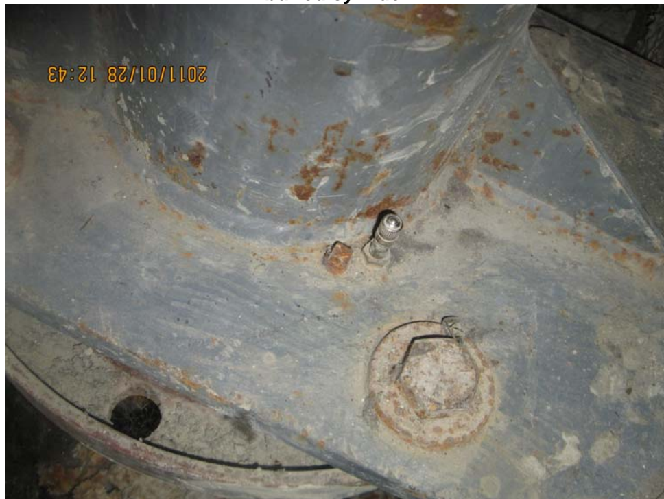
Photo 14 – Air valve and plug on jack flange for pressurizing plastic sleeve jacketing buried cylinder
