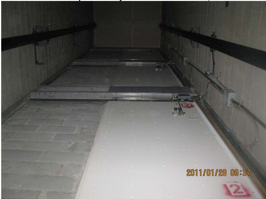
Photo 10 – Top of hoistway and entrances of floors 2, 3 and 4
