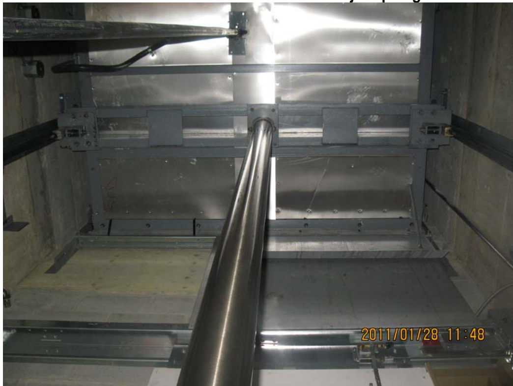
Photo 12 – Bottom of elevator car and jack plunger
