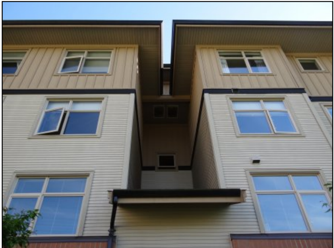
View of typical exterior cladding - Comprised of wood & batten siding, vinyl siding and brick veneer.
